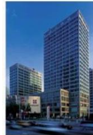
Concrete-filled steel tube structure: Ruifeng International: Business Plaza
