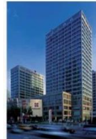
Concrete-filled steel tube structure: Ruifeng International: Business Plaza
