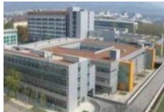
Accident & Emergency Hospital Linz
