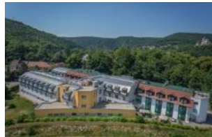
Rehabilitation Center Gars am Kamp
